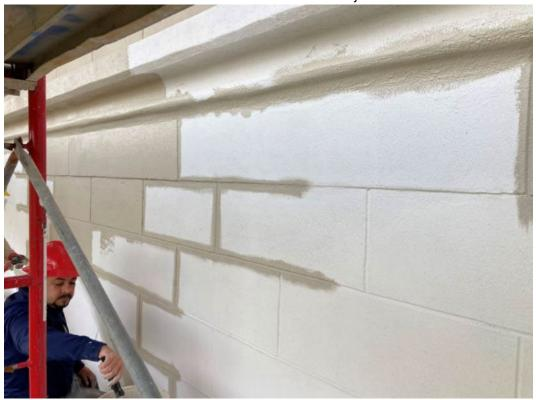
Three stages of paint work on the project. 30 year old paint ready to be primed on the bottom, white primer in the middle, finished paint topcoat on top, and to the right.
