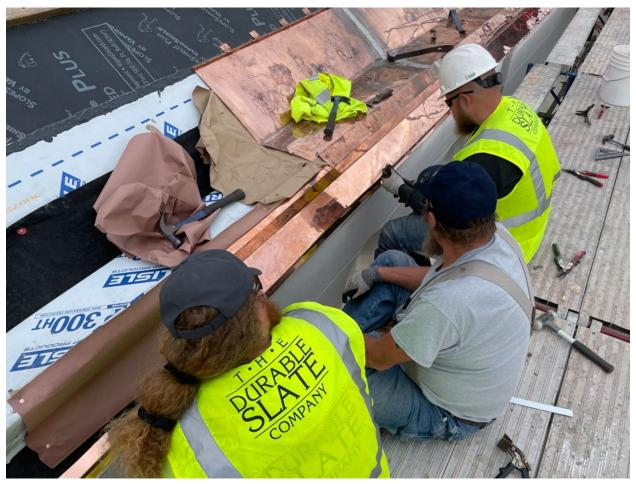
The hanging gutter on the east has been installed. Copper roofing metal specialists are soldering connections at the seams of the gutter and the downspout outlet tubes.
