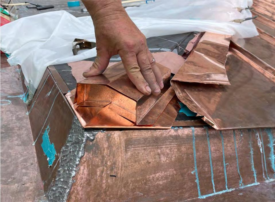
To ensure the roof copper is electrically grounded, properly bonded copper strips are being placed under the standing seam roof, passing through the roof deck at key locations.
