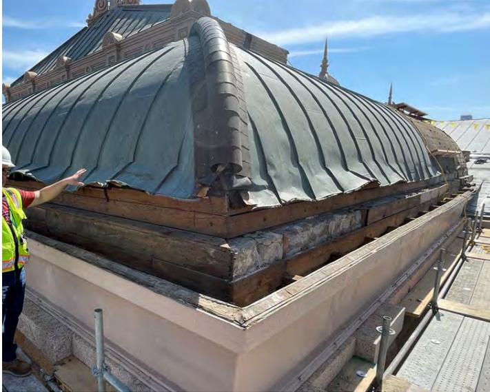
The opportunity is being taken to improve uplift resistance on the structure, which currently is 1888 wood framing in rubble limestone masonry.
